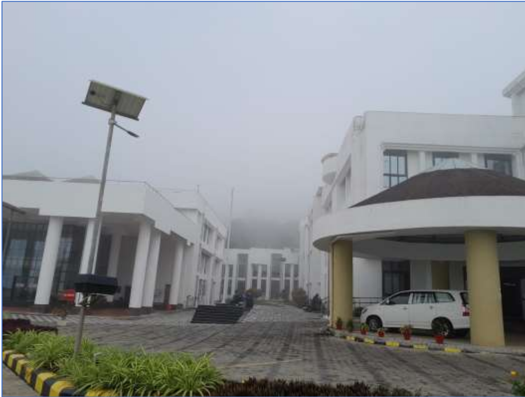
Fog: Open Cafeteria between Academic Block and Administrative Block
