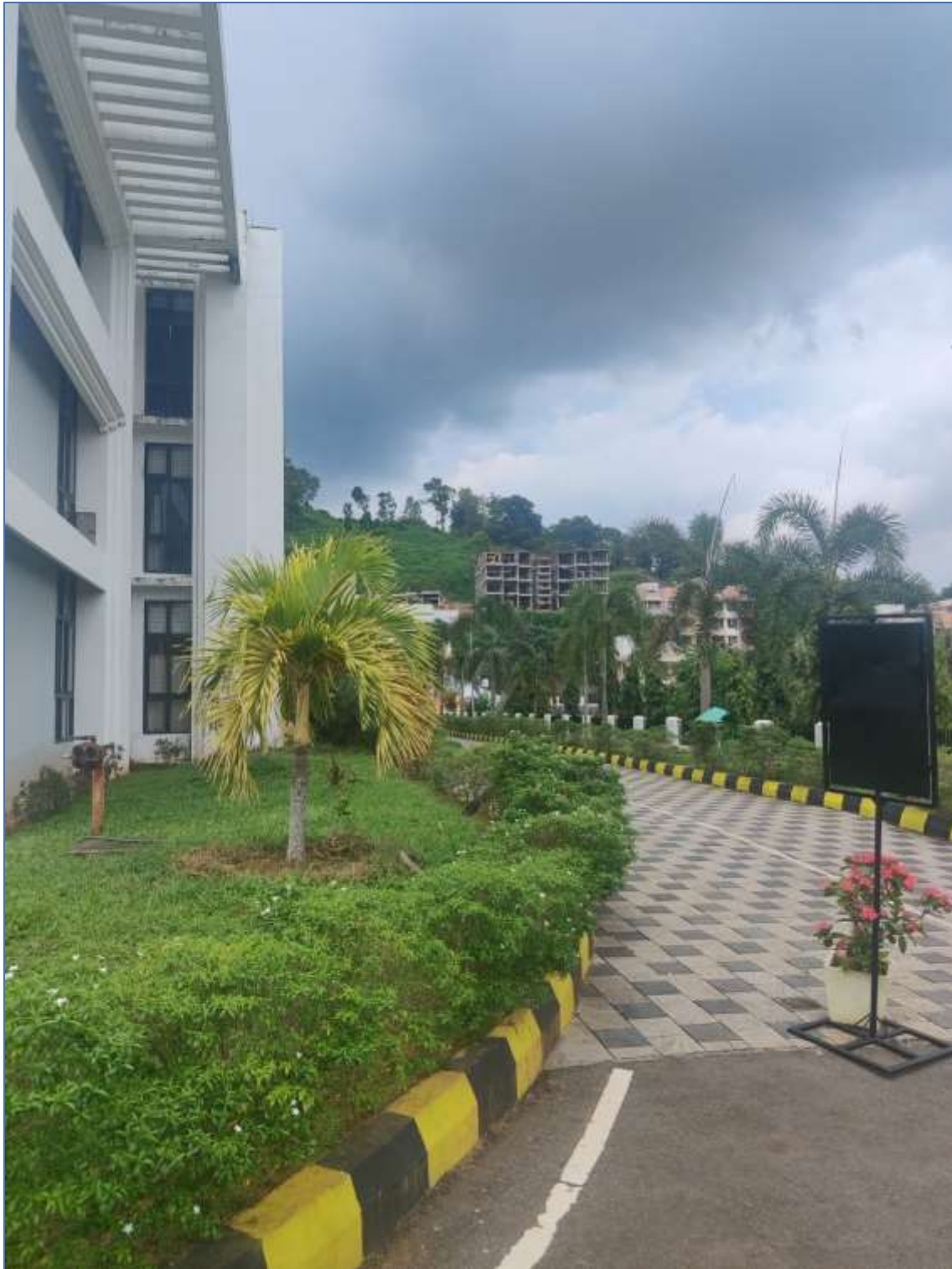
28 Staff Quarters Long Distance View Both the Buildings– Under Construction – Through Internal Revenue Generation (IRG) (on 02 Oct 2023)
