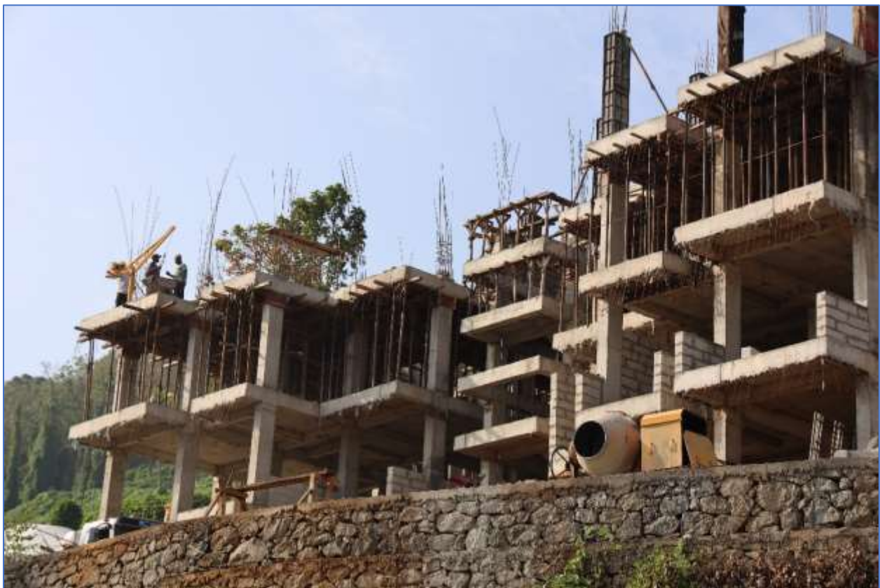
28 Staff Quarters 1 st Building – Under Construction – Through Internal Revenue Generation (IRG) (on 05 Feb 2024)
